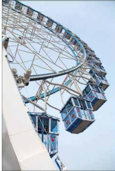
the conventional 8, providing greater transparency and an elegant structural appearance. Special v-shaped gondola hanging arms provide an excellent vista for all passengers.
